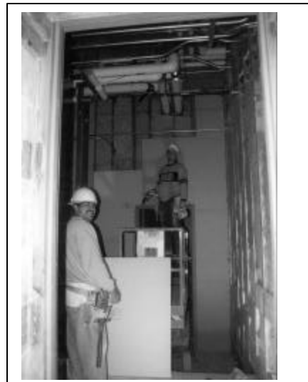
Figure 8. When visiting the construction site, we talked to subcontractors, and to Findorff workers (such as these workers installing drywall) about recycling. May 2003.
