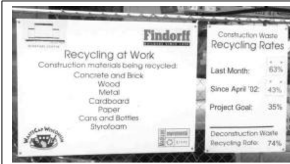
Figure 12. Three sets of signs were placed at the corners of the construction site in downtown Madison, October 2002.
