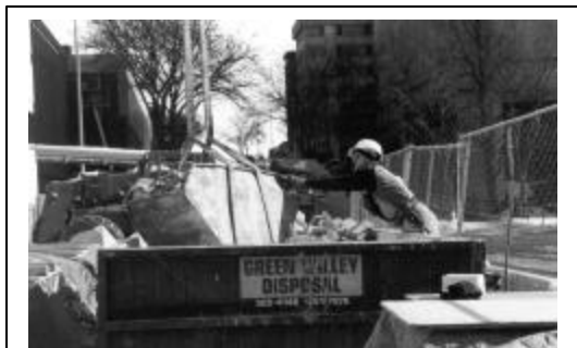
Figure 10. Recyclable materials, such as concrete, were collected in 1-yard carts throughout the construction site, and transferred to dumpsters. March 2003.
