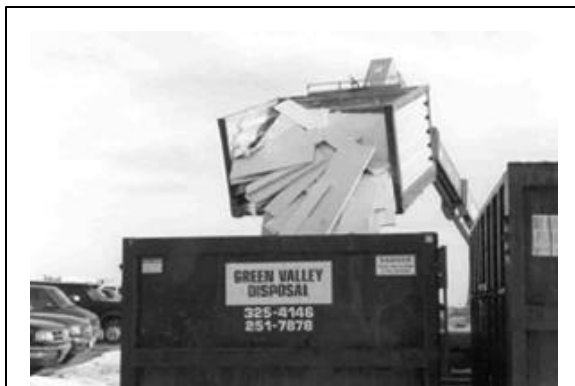
Figure 6. Drywall is dumped from a one-yard dock cart into a 20-yard recycling collection dumpster.
