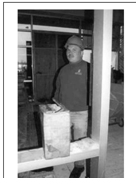
Figure 3. A subcontractor from Lurie Glass installing windows
