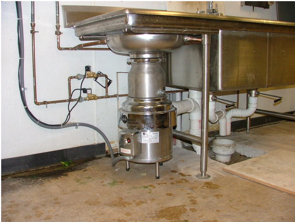
KINNICKINNIC DISPOSER INSTALLATION
