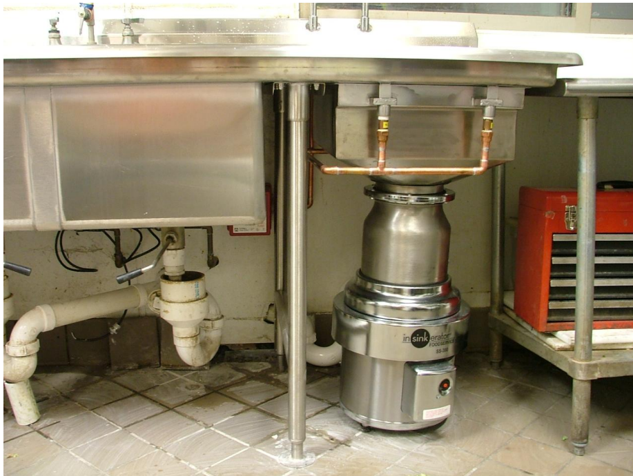
STATE STREET DISPOSER INSTALLATION
