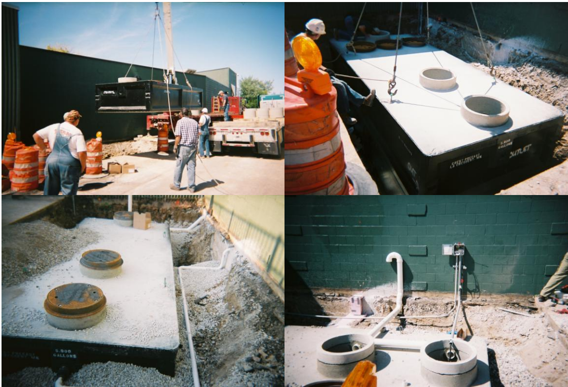
KINNICKINNIC SLURRY TANK INSTALLATION
